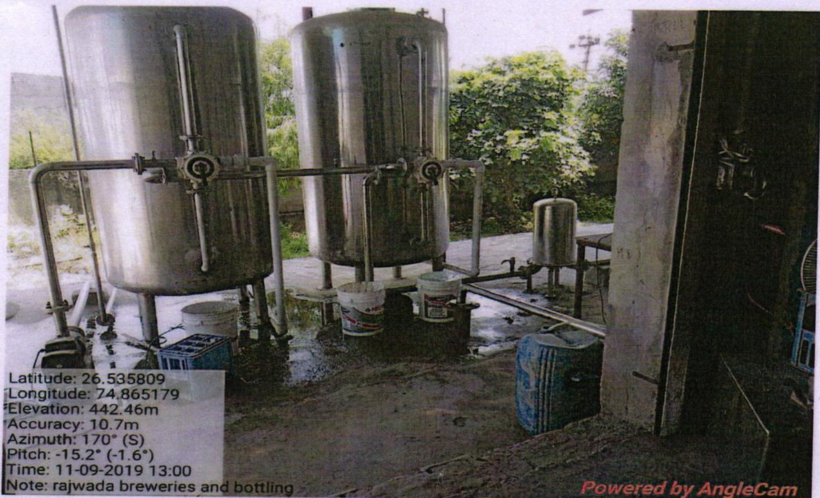
Filtration system (Sand and Activated Carbon Filter)
